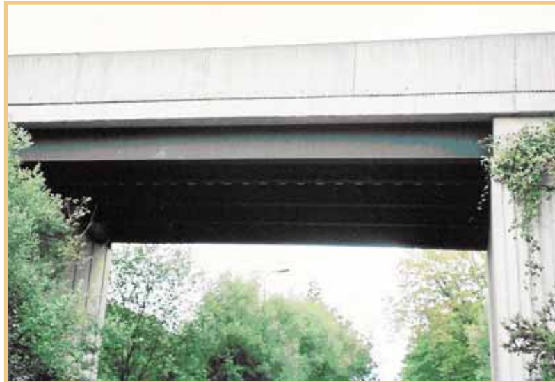
Figure 2.3 Bridge having weathering steel beams
