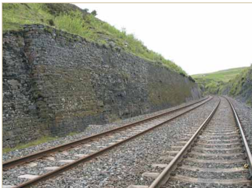
Figure 1.3 Drystone retaining wall, Settle – Carlisle Railway Line (courtesy Mouchel)
