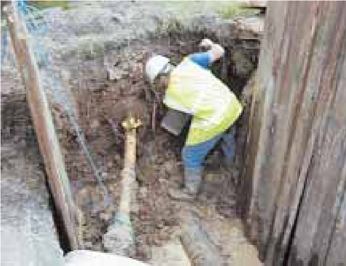
Water that has collected in trenches may have become stagnant and infected
